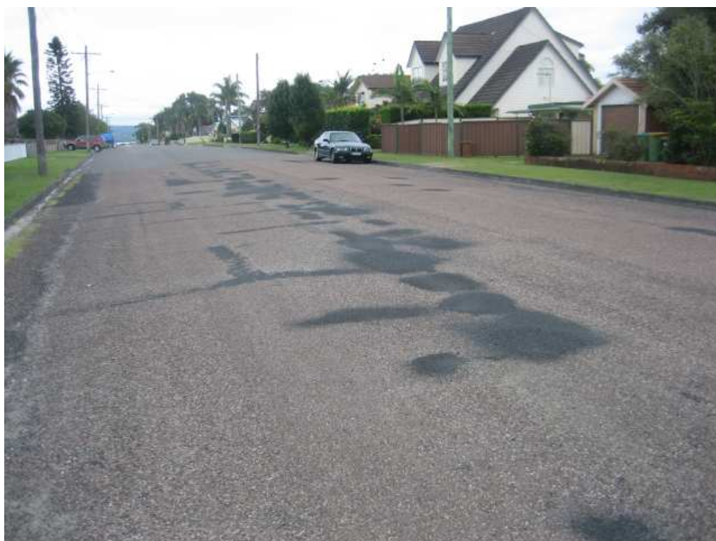
PACIFIC STREET LONG JETTY
